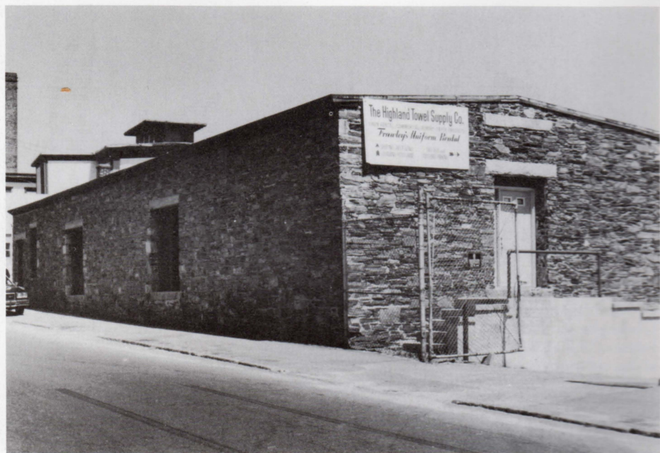
24. Richmond Mill Storehouse, Lawrence St., ca. 1850. The Concord River was exploited for water power even before the textile mills were established in the 1820s. This rubblestone building was the storehouse for Richmond's paper and cotton batting mill. Note that although the rubblestone is carefully laid in horizontal courses along the front of the building, the sides and rear are constructed of randomly laid stone. Nearby, at 224, 228 and 310-326 Lawrence St., are dwellings built to house some of the mill's employees.
